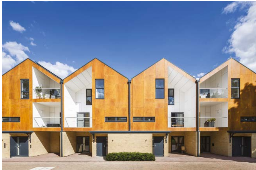
Woodview Mews – Croydon, UK – Geraghty Taylor Architects
