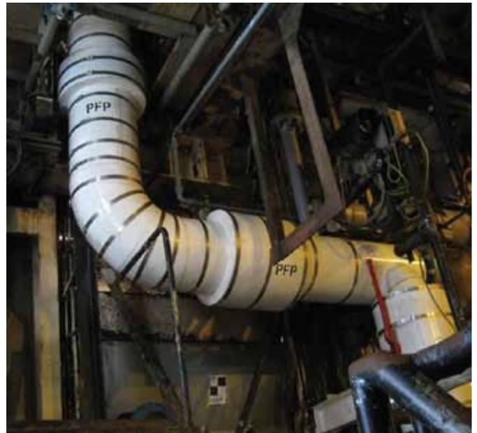
FOAMGLAS® XP: up to two hours of jet-fire resistance
