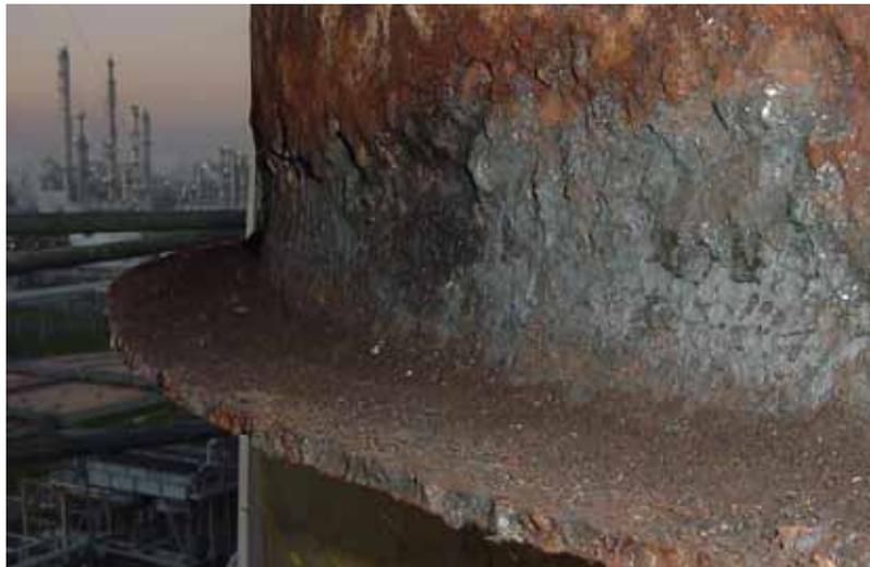
When an insulation material is wet, it may never fully dry out. When insulation remains wet, it does not perform as advertised, a costly consequence to the owner.
