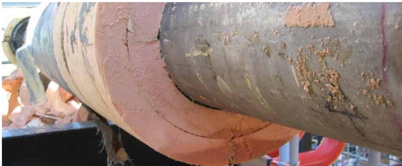
Dismantling of wet PU before replacing it with new dry FOAMGLAS® Insulation at an UK gas plant
