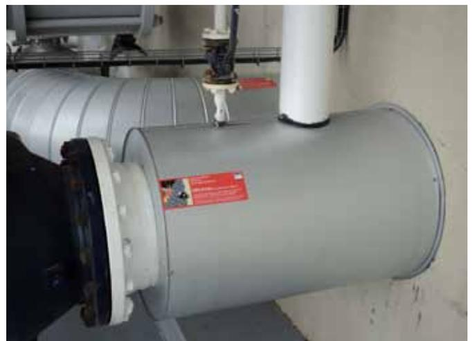
*Fire resistance for fire-wall pipe penetrations*
